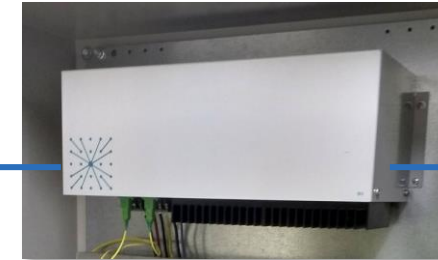
Passive current sensor modules (three-phase, secondary-connected)
