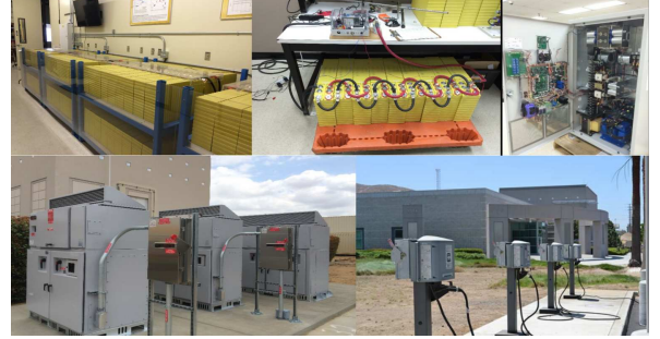
Fig. 1. The energy resources at the University of California at Riverside's CE-CERT microgrid. From left to right and top to bottom: battery racks, battery connections, battery inverter, solar panel inverters, and EV chargers.
