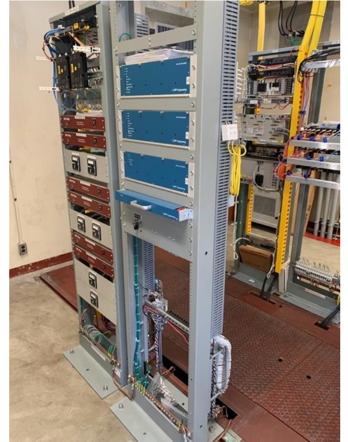
Digital fault recorder at a distribution substation Photo courtesy of Southern California Edison
