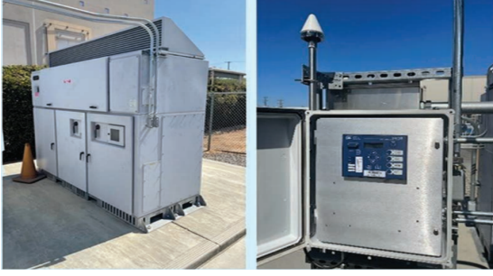
Fig. 1. A WMU installation at an IBR: (left) a three-phase commercial PV inverter; (right) a WMU to record GPS time-stamped waveform measurements.
